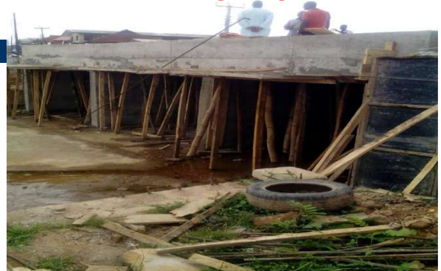
Above represents sample of parts of the on-going work at the site
