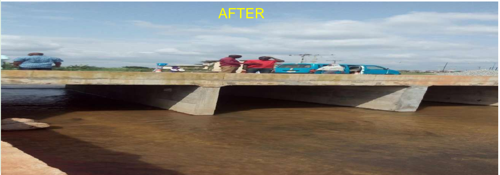
Above represents sample of parts of the completed work
