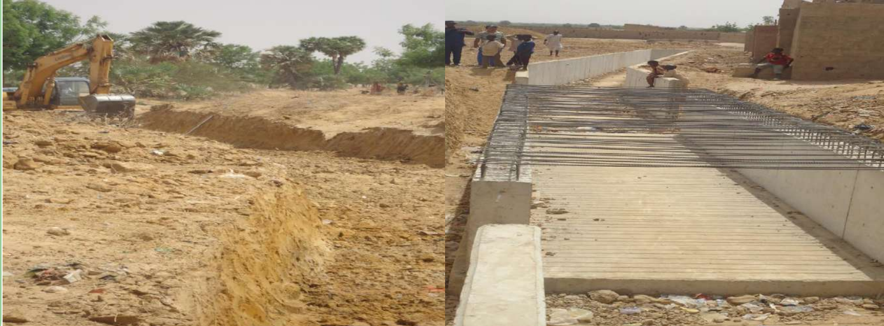
Above represents sample of parts of the on-going work at the site
