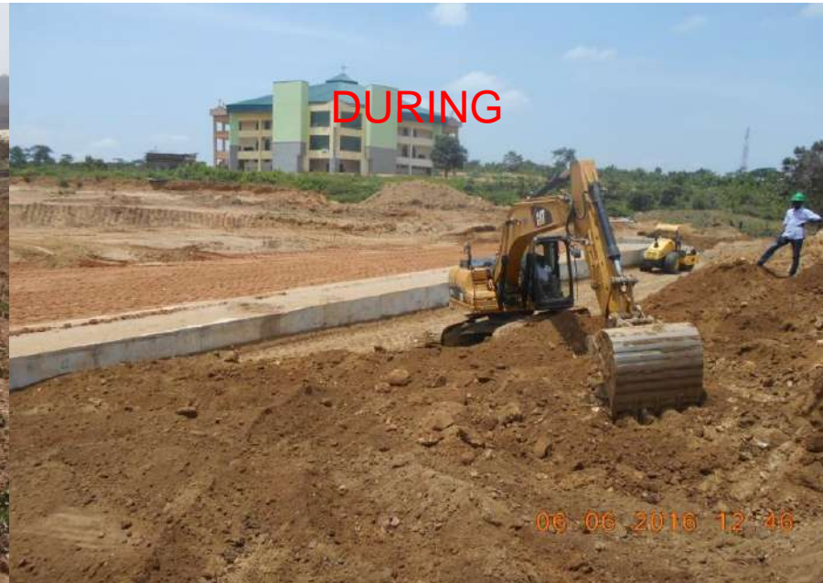
Above represents sample of parts of the on-going work at the site
