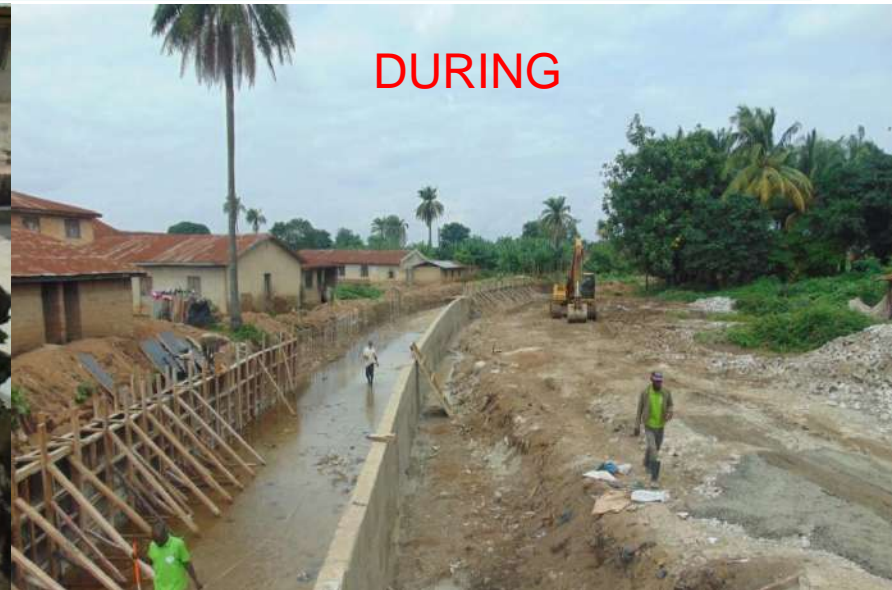
Above represents sample of parts of the on-going work at the site
