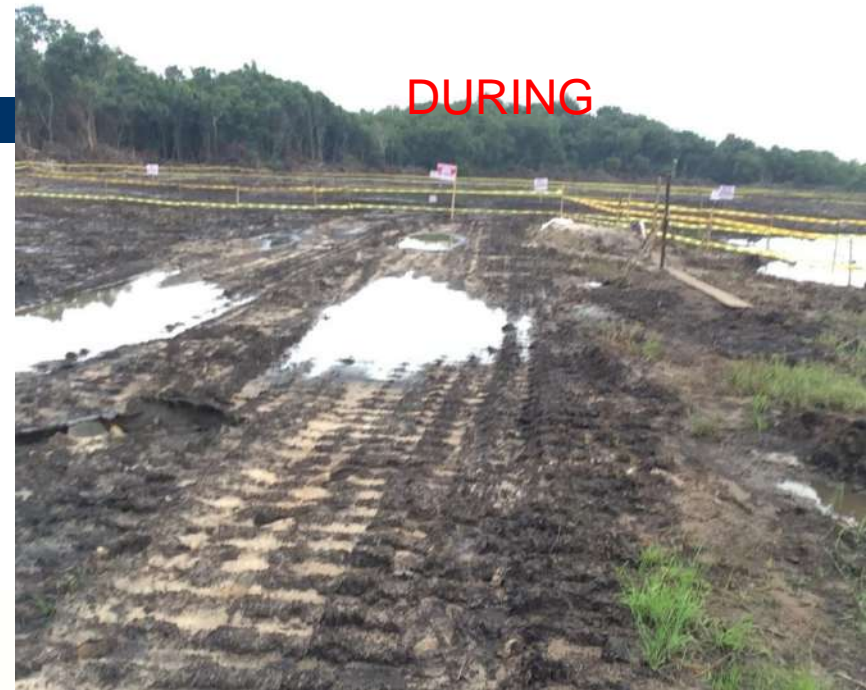
Above represents sample of parts of the on-going work at the site
