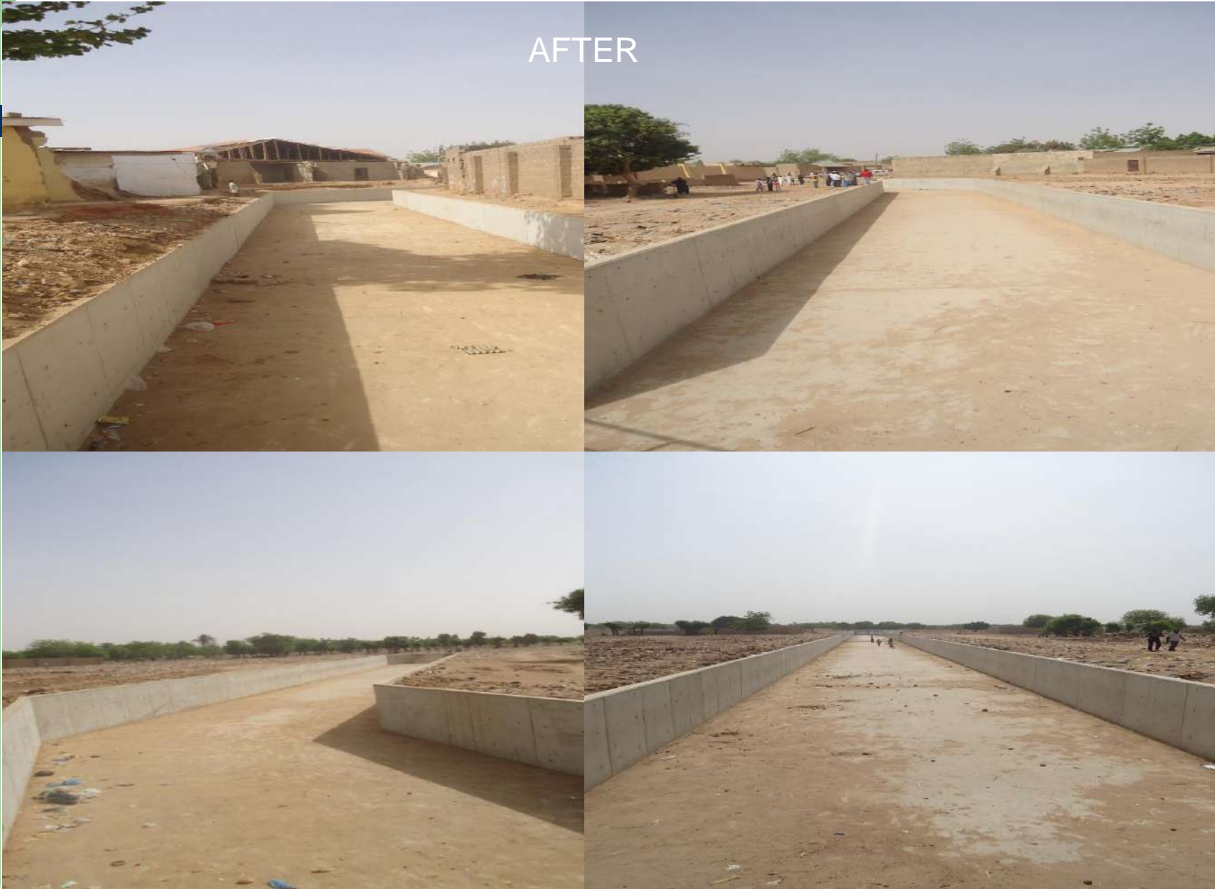
Above represents sample of parts of the completed work
